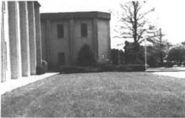
BEFORE: The front of the building is dominated by mown lawn and a few masses of evergreen trees and shrubs. U.S. Fish and Wildlife Service Building Annapolis, Maryland
